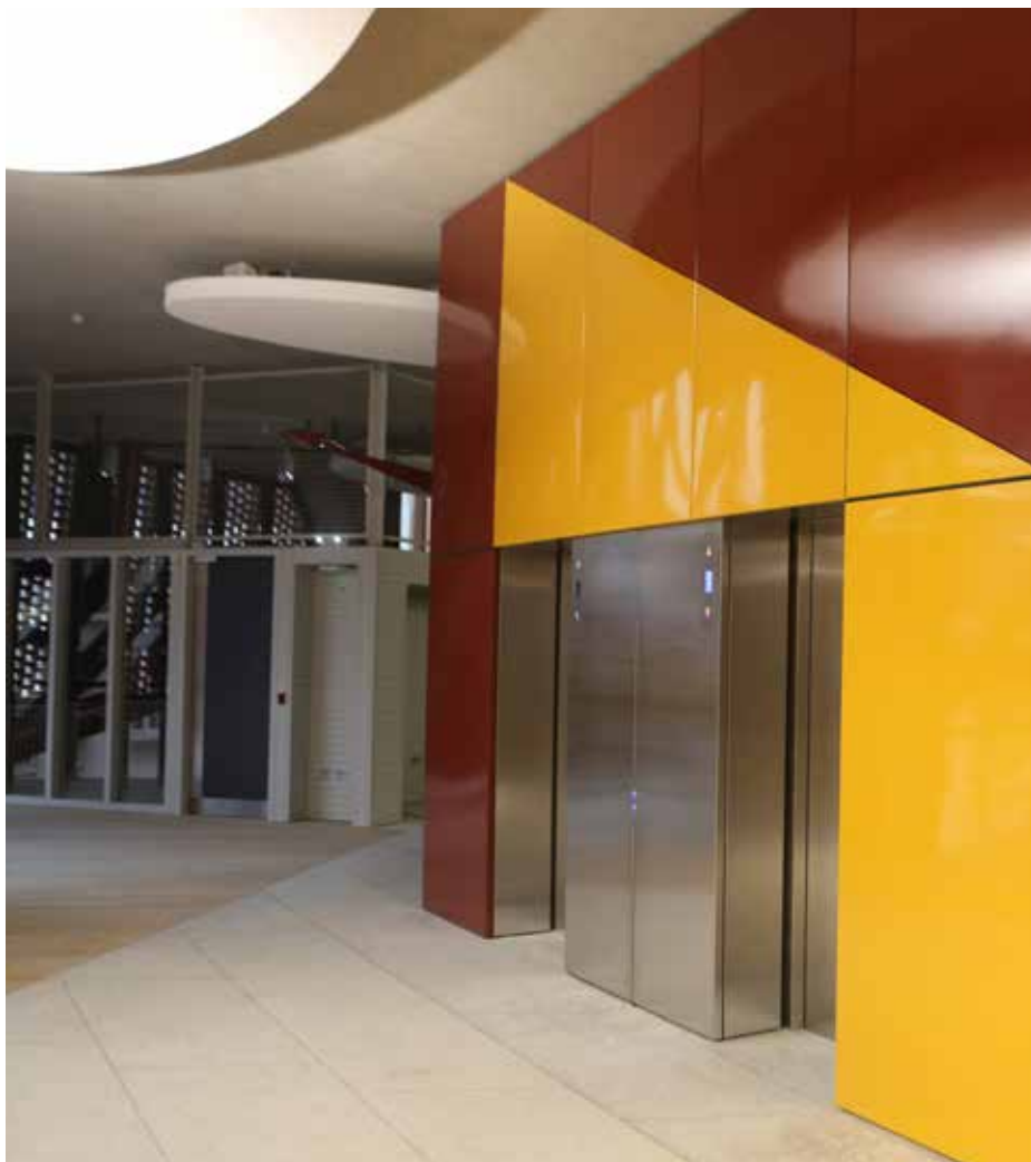
The London School of Economics' Saw Swee Hock Student Centre – Multi-coloured Vitreous Enamel wall linings installed by SAS Project Management. Architect – Twomey Architects.
