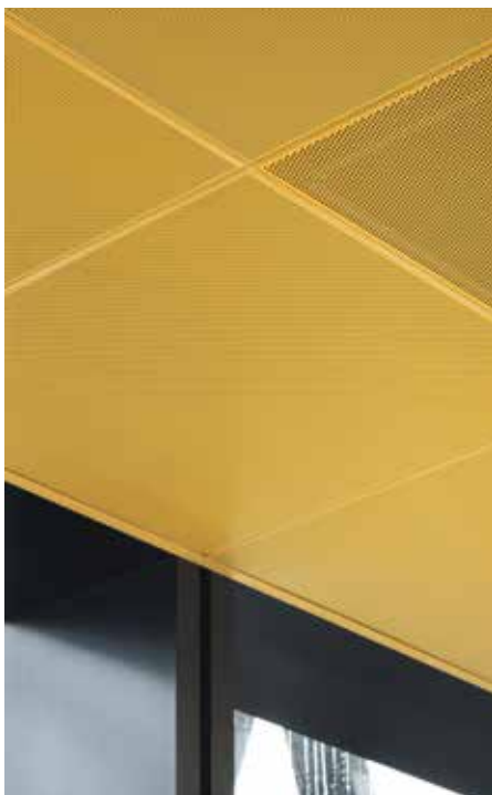
Library of Birmingham – System 150 finished in Strontium Gold (see case study on page 18-19 of this Insider). Architect – Mecanoo.
