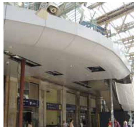
Waterloo Station London - Phase 3
