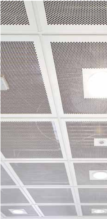
Howberry Business Park, Wallingford Chilled Beams, Room Comfort
