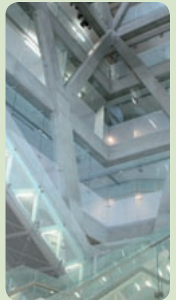
Monsoon – Atrium Glazing
