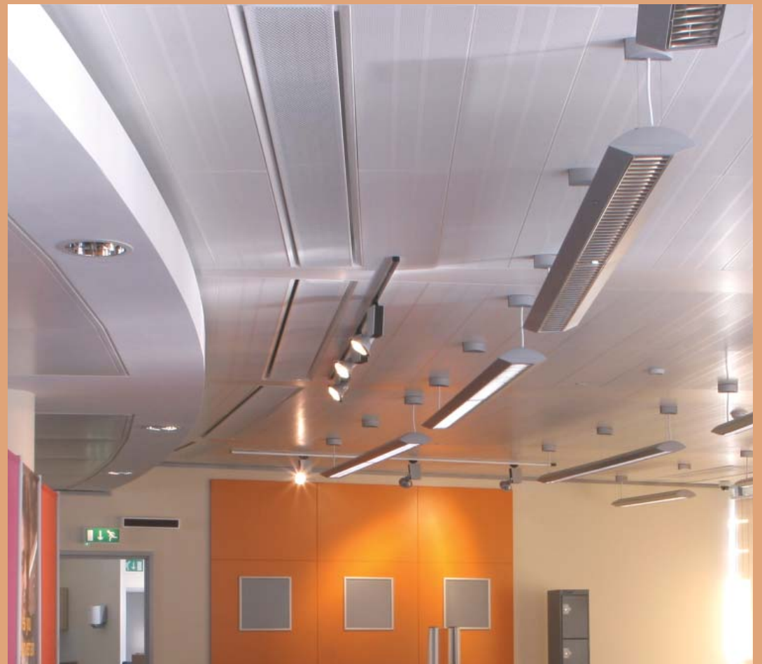
Active Chilled Beams provide comfort cooling
