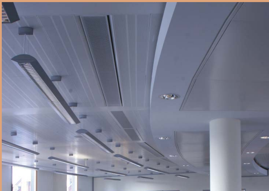
Active Chilled Beams in radial building
