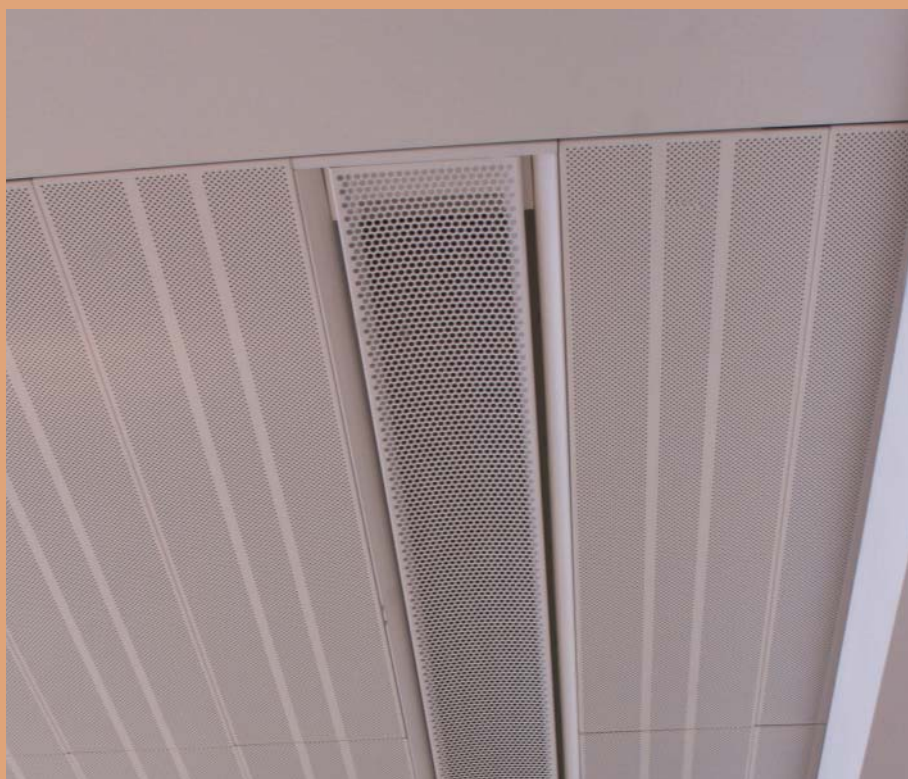
Active Chilled beam integrating with SAS metal ceiling
