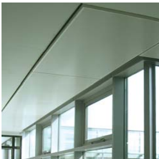
Radiant heating panels
