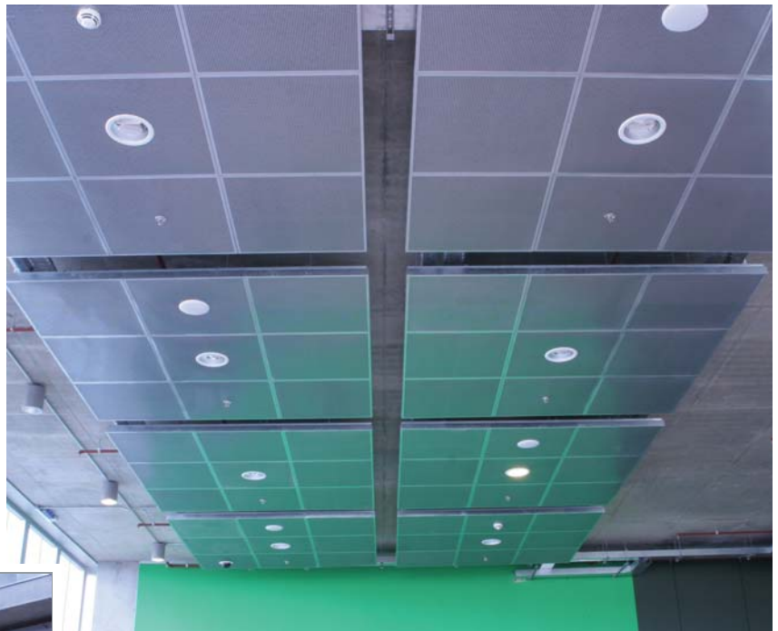
System 600 rafts feature in the atrium ceiling
