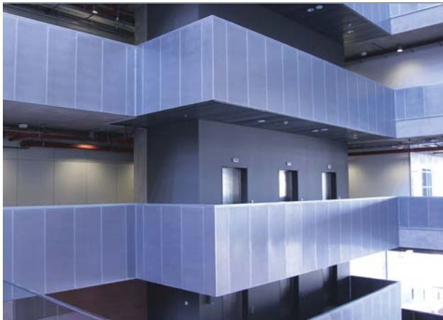
Clear finish galvanised wall panels are used throughout the building
