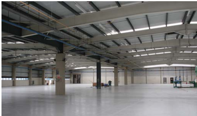
Interior of new Bridgend building
