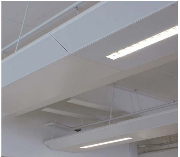
Modules feature SAS System 600 and HCP radiant heating panels
