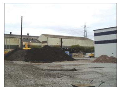
Work has already started on site at Apollo Park
