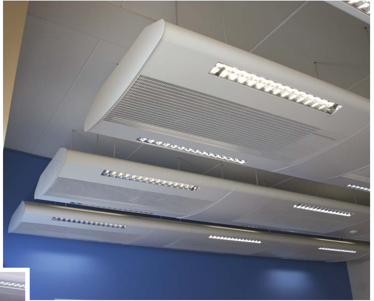
ISMs featuring both up- and down-lighting
